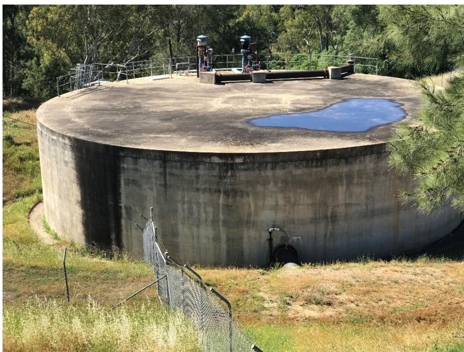
Source: Atom Consulting, taken October 2016
