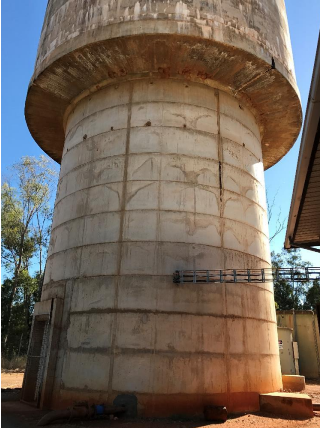
Figure 15-3 Mt Arthur – Ganmain high level reservoir
