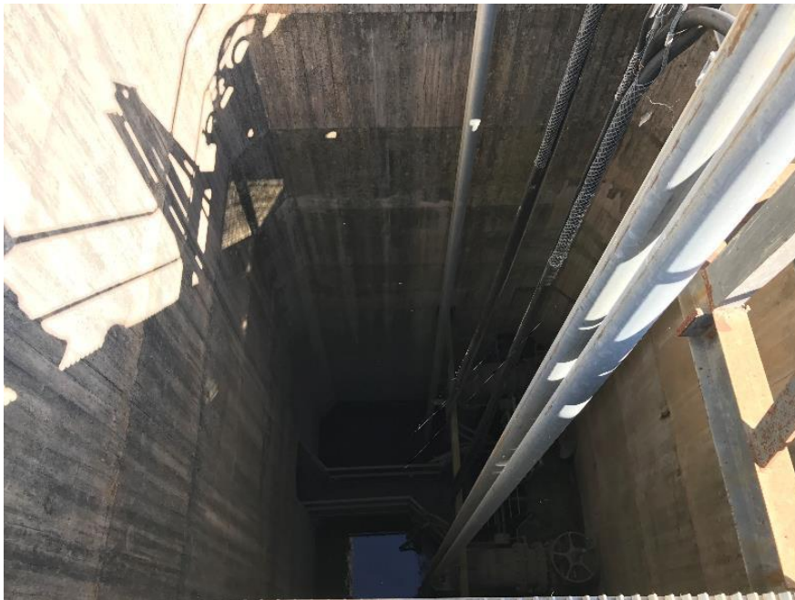
Figure 4.2 Murrumbidgee River Extraction Point
