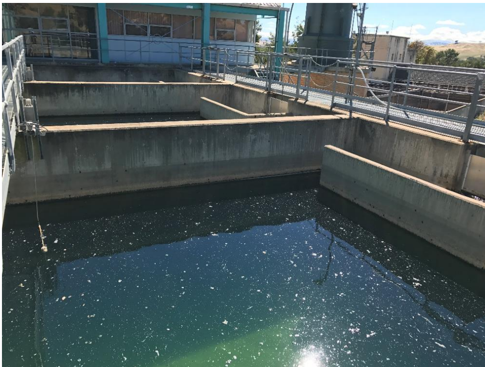
Figure 13-4 Jugiong Water Treatment Plant - Filters
