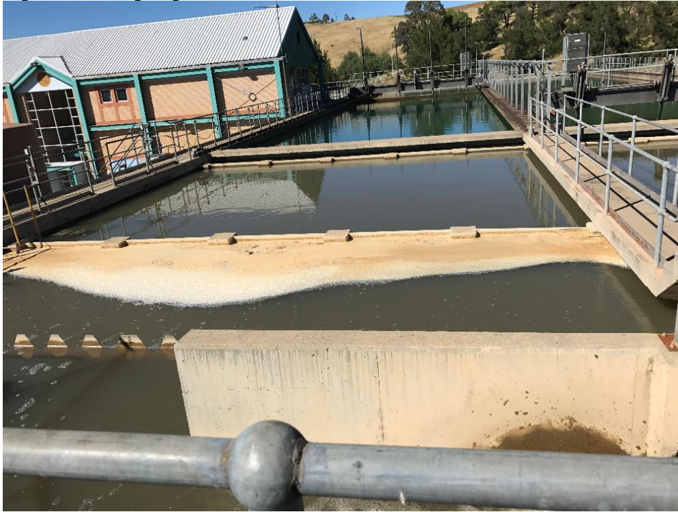
Figure 13-3 Jugiong Water Treatment Plant - Clarification
